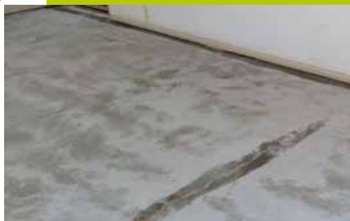
Garage floor crack repair
